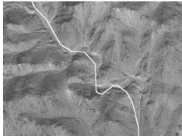
Figure 23: ITD drainage feature.
